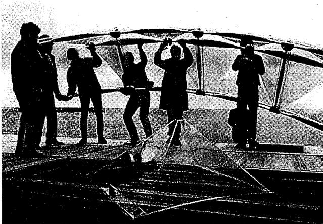
Fig. 1. Renzo Piano Building Workshop, IBM Traveling Pavilion, erection of system. (Courtesy of Renzo Piano Building Workshop.)
