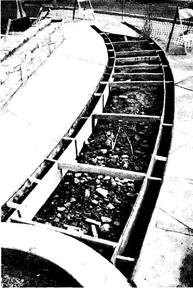
Fig. 8. Formwork during construction of the concrete rails.
