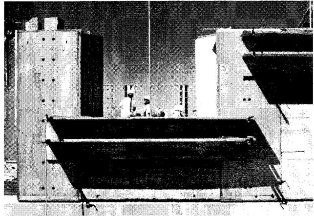
Fig.1 Incremental formwork for classroom facility
