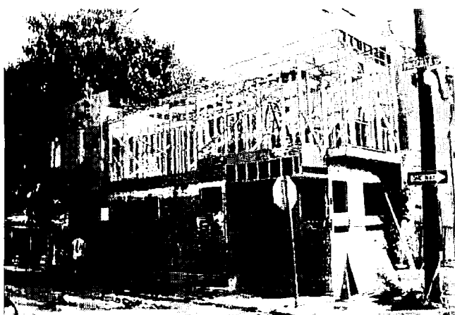
Fig. 1. Rowhouse under construction.
