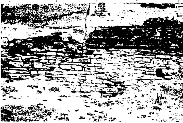
"Retaining Wall, East Liberty".
