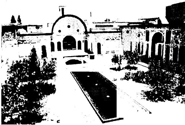
Fig. 4. Tabataba'i House: view from the courtyard.
