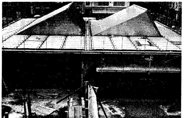
Fig. 5. The Brancusi Workshop: glazed roof under construction.
