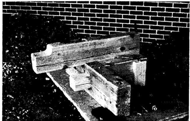
Fig. 3. Gamble House beams with additional pad attachment.
