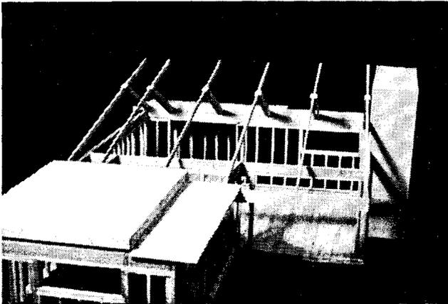
Fig 4. R.M. Schindler, Felix Presburger House, Studio City 1945-47. Framing model, scale 1"=1'-0", constructed by DalTech students July 1998.
