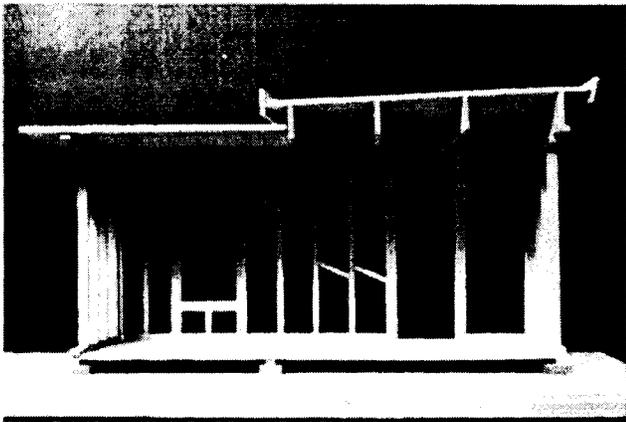
Fig.2. Schindler Frame sampler model, scale 1"=1'-0", constructed by DalTech students July 1998.
