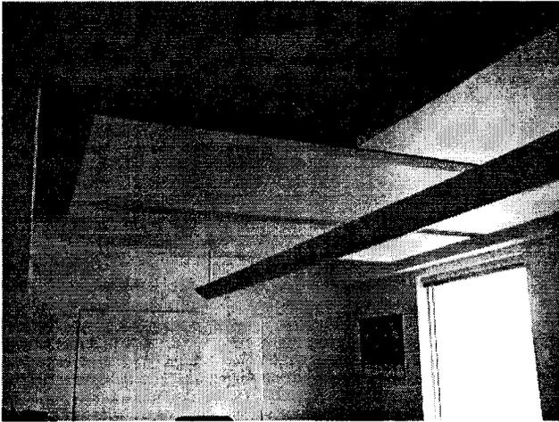
Fig. 3 View of ceiling showing radiant heating panels
