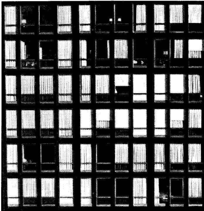
Fig. 3. 860-880 Lake Shore Drive, Chicago; Ludwig Mies van der Rohe, 1951. An elevational richness generated by the ambiguity between frame/infill and space/skin relationships.
