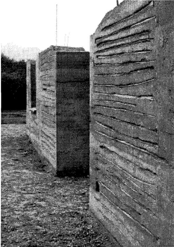
Fig. 6. Completed rammed earth walls of Gila dwelling with saguaro cactus ribs
