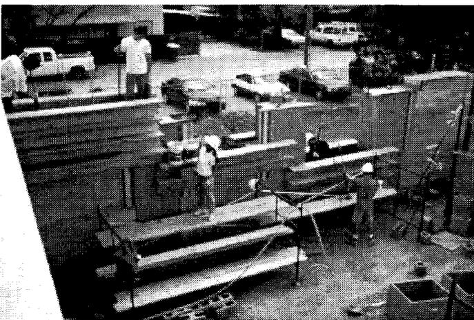
Fig. 2. Staggered wall forms system for classroom building.
