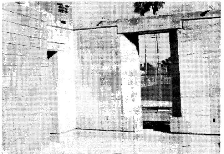
Fig. 4. Completed rammed earth walls with forms removed
