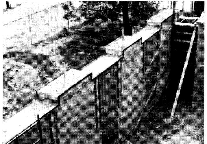
Fig. 3. Tamped rammed earth walls
