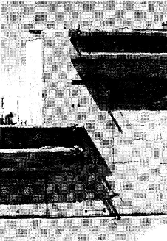
Fig. 1. Plywood and pipe clamps forms for classroom facility.
