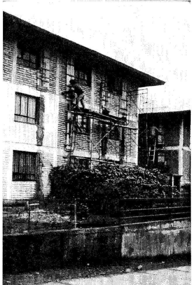
Fig 2. Seismic strengthening of concrete frame and shear wall
