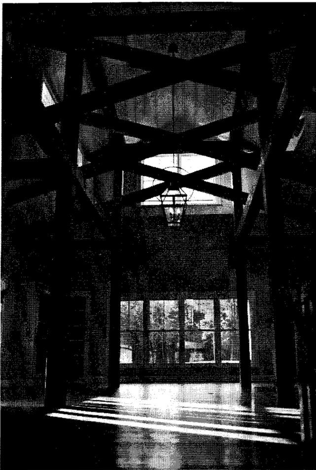
*Fig. 4. Living room truss made from recycled timbers.*
