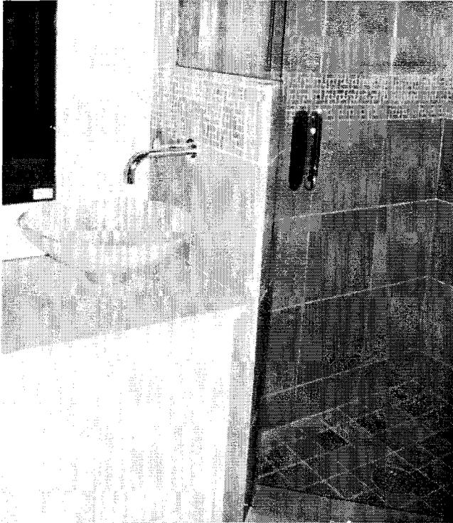
*Fig. 5. Stone tiled shower set with thick set mortar and sanded grout.*
