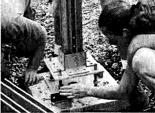
*Fig. 7. Moveable foundation pads and leveling screws for the transformable structure.*
