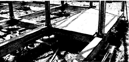
*Fig. 9. Beams and columns serve as a utility grid and to support the floor inserts*
