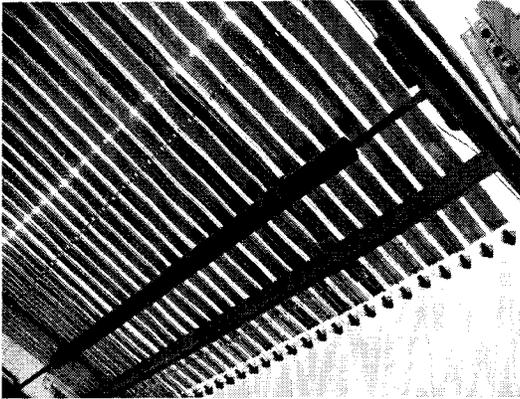
Fig. 15. Evacuated tube solar hot water heater.
