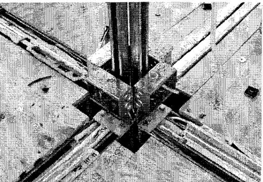
*Fig. 9: B-Line recycled steel columns and beams are bolted together to form an open building system.*
