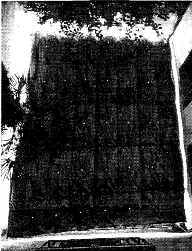
Fig. 7. The translucent toldo diffuses sunlight, and absorbs less heat than the darker opaque version. Bornos, Spain, Calle Alta. From John S. Reynolds, *Courtyards: Aesthetic, Social, and Thermal Delight* (New York: John Wiley and Sons, 2002; page 144.)
