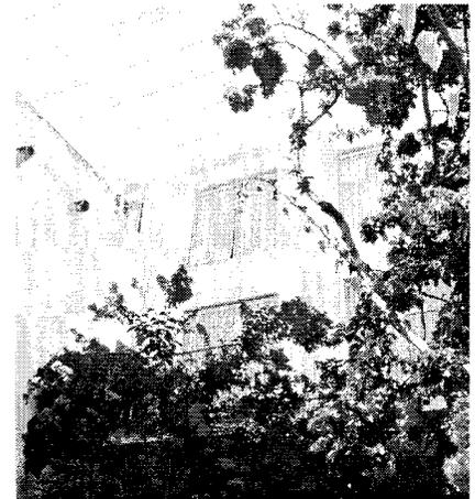
Fig. 6. The nearly opaque *toldo* darkens the courtyard by day, protecting everything below from direct sun. The small holes prevent accumulated rain from adding unsupportable weight. Cordoba, Spain, Calle Osio. From John S. Reynolds, *Courtyards: Aesthetic, Social, and Thermal Delight* (New York: John Wiley and Sons, 2002; page 87.)
