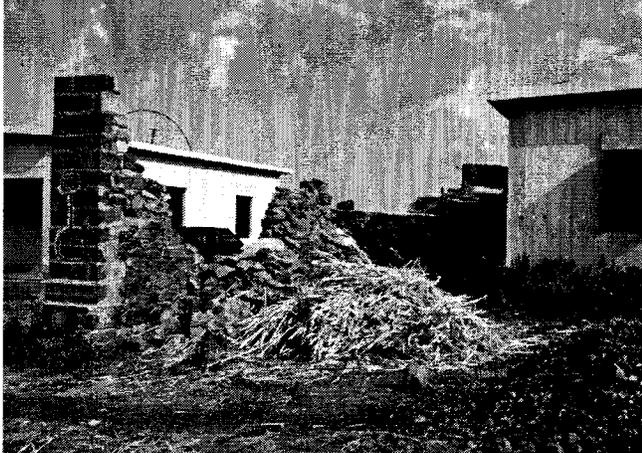
*Fig. 8. Newly built wall that collapsed after only 2 monsoon seasons, new Sirsal, 1996. Photo courtesy of Rajendra Desai.*
