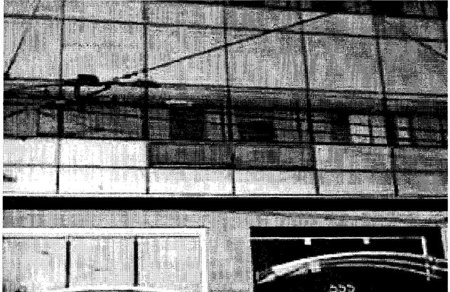
Fig. 8. Here we can see the differentiated glazing: clear versus fritted glass, and two of the operable windows in an open position.
