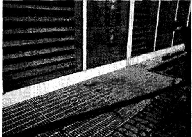
Fig. 4. View of air intake grille at base of building. Note clouding on center glazed unit.
