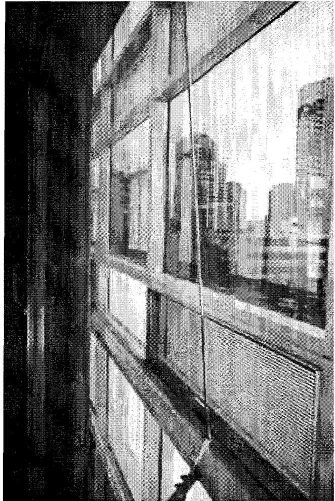
Fig. 14. View looking into the cavity. Note the differentiated glazing materials: clear and fritted, as well as the operable window.
