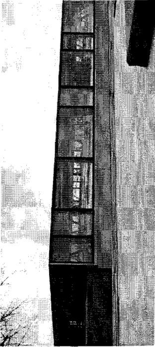
*Fig. 16. A view of the side elevation of the attached double skin component. You can clearly see through the entire space and it is evident that the space is not compartmentalized. The structure that holds the curtain wall away from the existing concrete frame forms a lacelike network within the cavity.*
