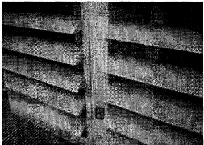
Fig. 5. It can be seen that the louvers are fixed in a horizontal position, painted white and are very dirty.
